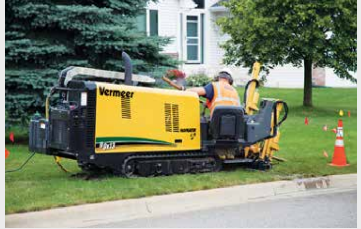
Trenchless - Horizontal Directional Drilling
