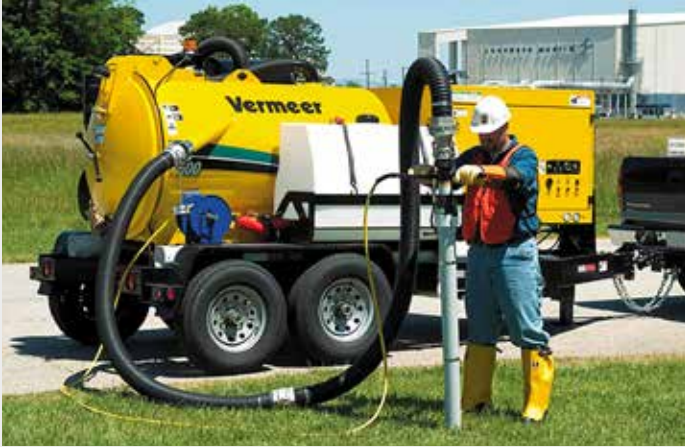
Hydro Suction Footing Excavation
