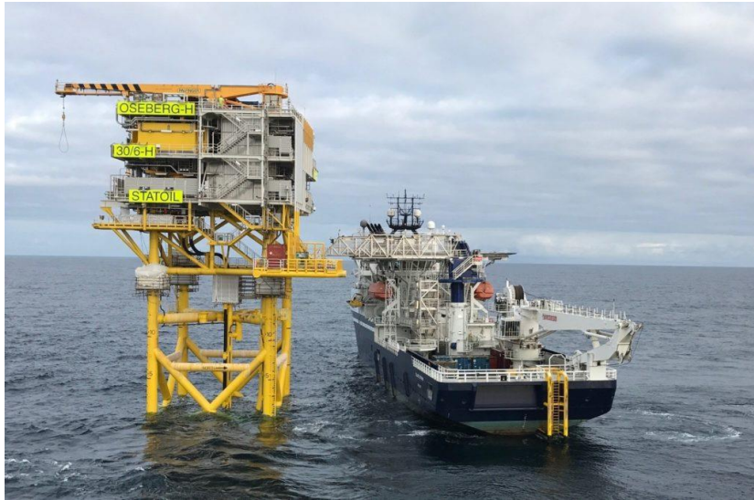
OIL AND GAS: Using service vessel to walk-to-work on an oil and gas installation
