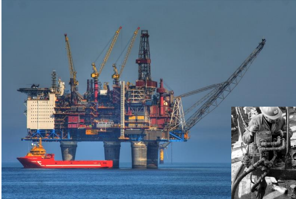
Gullfaks, picture by Statoil/Equinor
