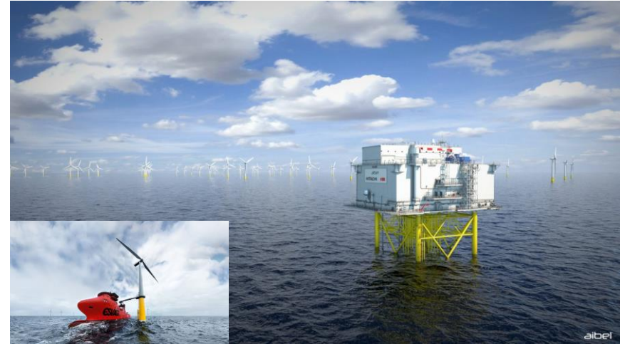
OFFSHORE WIND: High Voltage DC transformer Doggerbank (UK) with walk-to-work solution for both transformer and wind turbines
