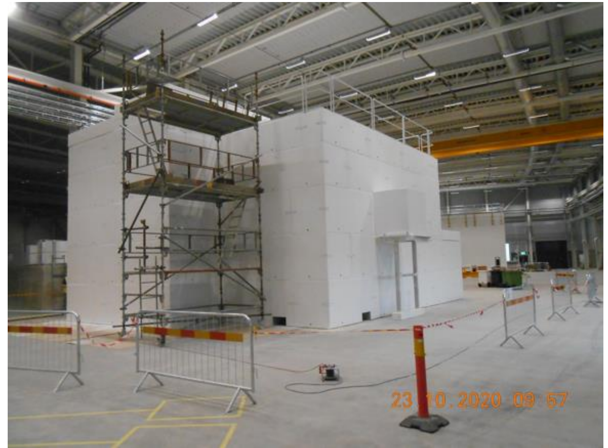
Bifrost cave completed construction
